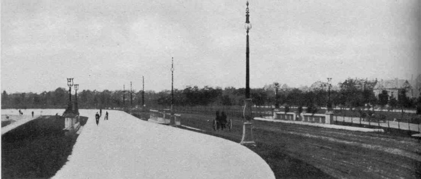
Garfield Park half-mile cement bicycle track, built in 1896
